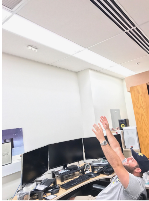
Figure 1: Michigan Computer Science & Engineering Ph.D. student Connor Bolton notices that an ultrasonic room occupancy sensor in the ceiling had been bathing his experiments with unwanted 25 kHz sounds.
